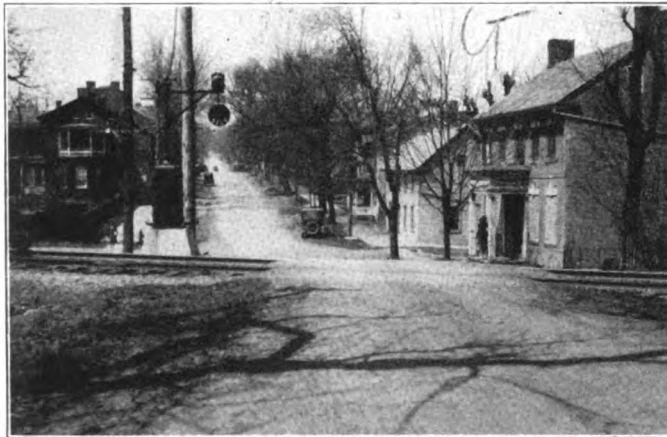
Typical Installation of 110-volt A. C. Magnetic Autoflag
