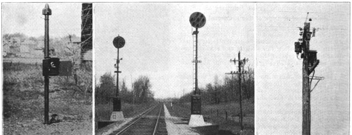
A Telephone Is Located at Each Passing Track
