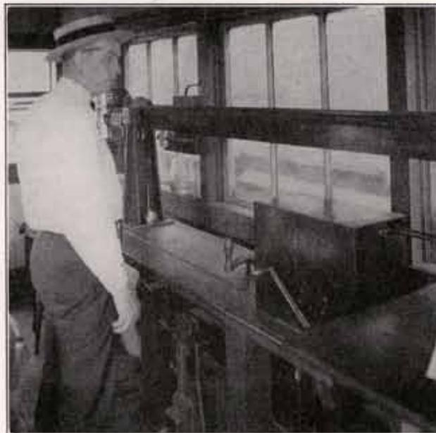
Fig. 2. Weighing a car with a Streeter-Amet recording attachment
