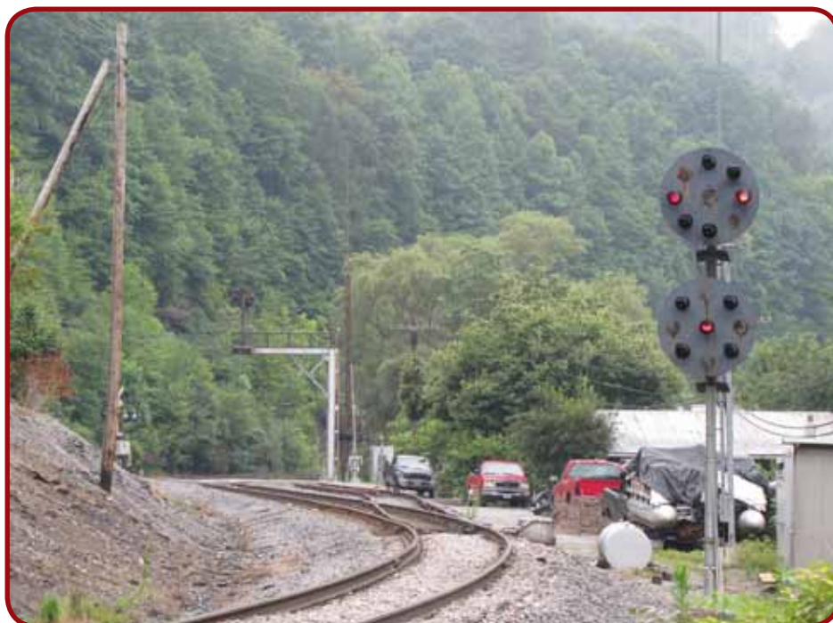
Lark, Virginia - Big Creek Branch - Clinch Valley District
