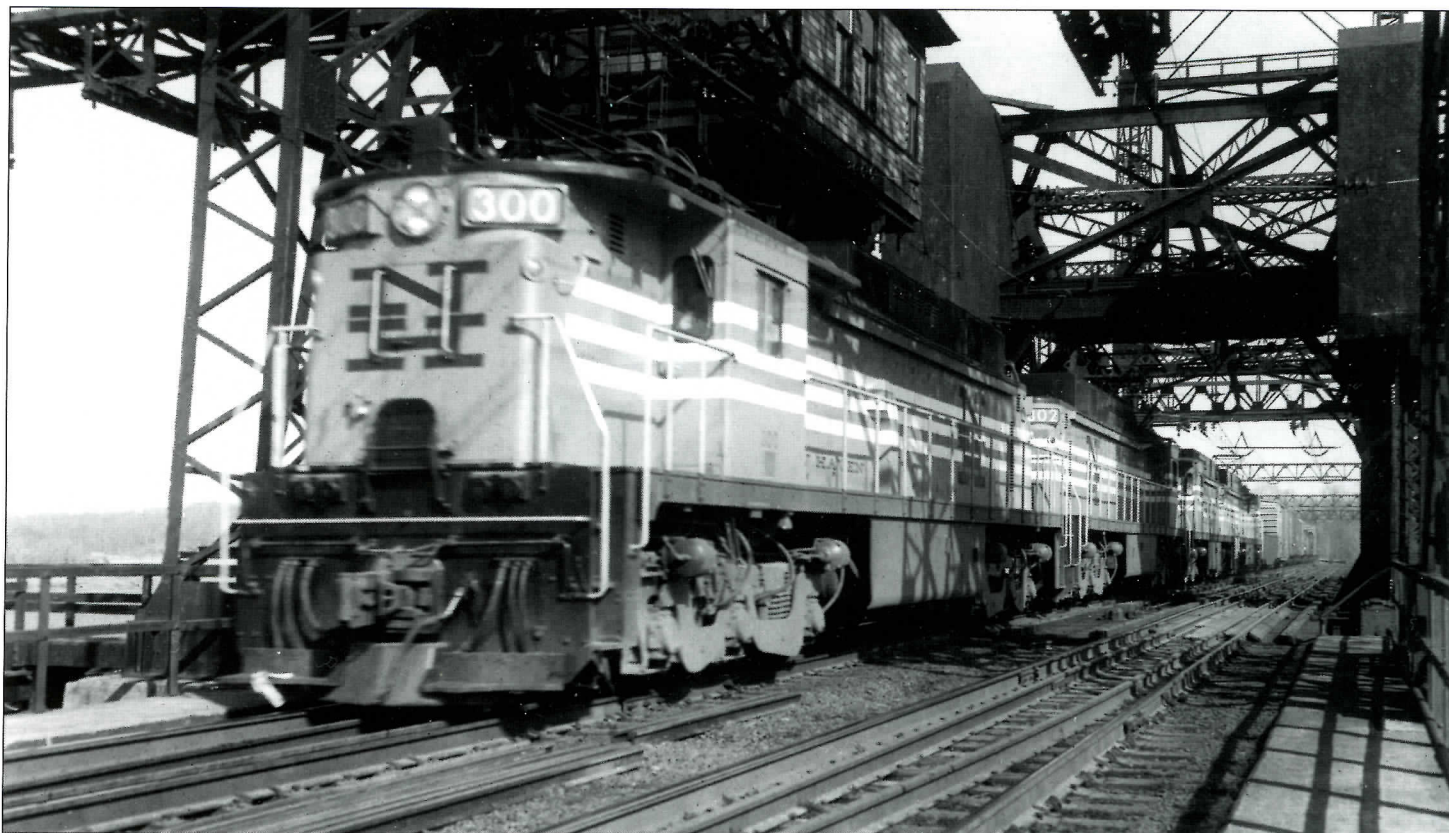
Above: Four EF-4s were required on this train due to a shortage of enough rectifier tubes which cost $4,350.00 each. NH #300, #302, #309 and #310 on NG-1 were photographed at S.S.14, Pelham Bay, New York on February 5, 1964. Photo by H. Goldsmith, J. W. Swanberg collection. Below: On September 17, 1966, fireman J. W. Swanberg took this photo at approximately 11:00 a.m. from the cab of New Haven U25B #2524 which was on the head end of OB-6 from Maybrook. New Haven #301 and #304 were on the freight seen below as it was ready to leave Cedar Hill with a New York bound freight. Photo by J. W. Swanberg.
