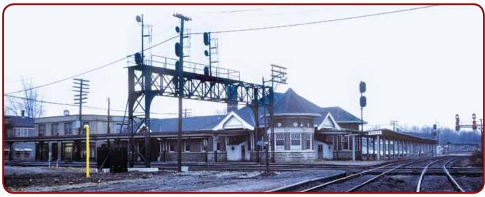
Dave Oroszi photographed the Marion Union Depot from the C&O tracks on the north side of the Erie-NYC tracks. The shed over the C&O side of the depot was built to a C&O design, hence the two posts supporting the structure. The Erie and NYC shed are the more usual single post and cantilever style. To the left of the depot is The Erie terminal building was located to the left of the depot.
